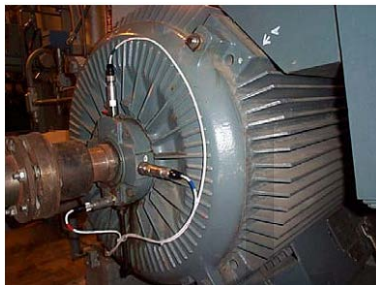
Fig:-Measuring Motor Bearing Vibration
